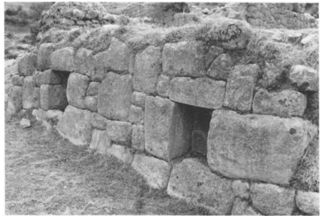
Fig. 13. Detail, niched terrace wall, Rumi Wasi (author).
