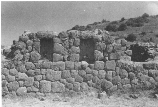
Fig. 12. Detail, west wall, Building 2, Rumi Wasi, showing niche frame and conspicuous mud mortar in the area between niches (author).
