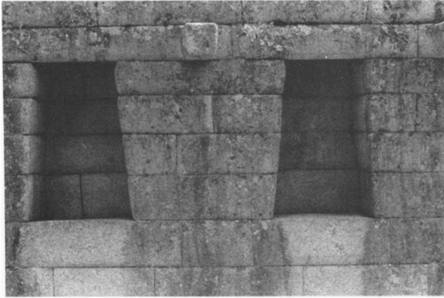
Fig. 19. Niched building interior, Machu Picchu (author).
