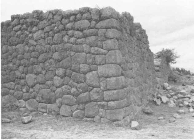
Fig. 15. Detail, exterior building corner, Rumi Wasi, Building 1, front wall (author).
