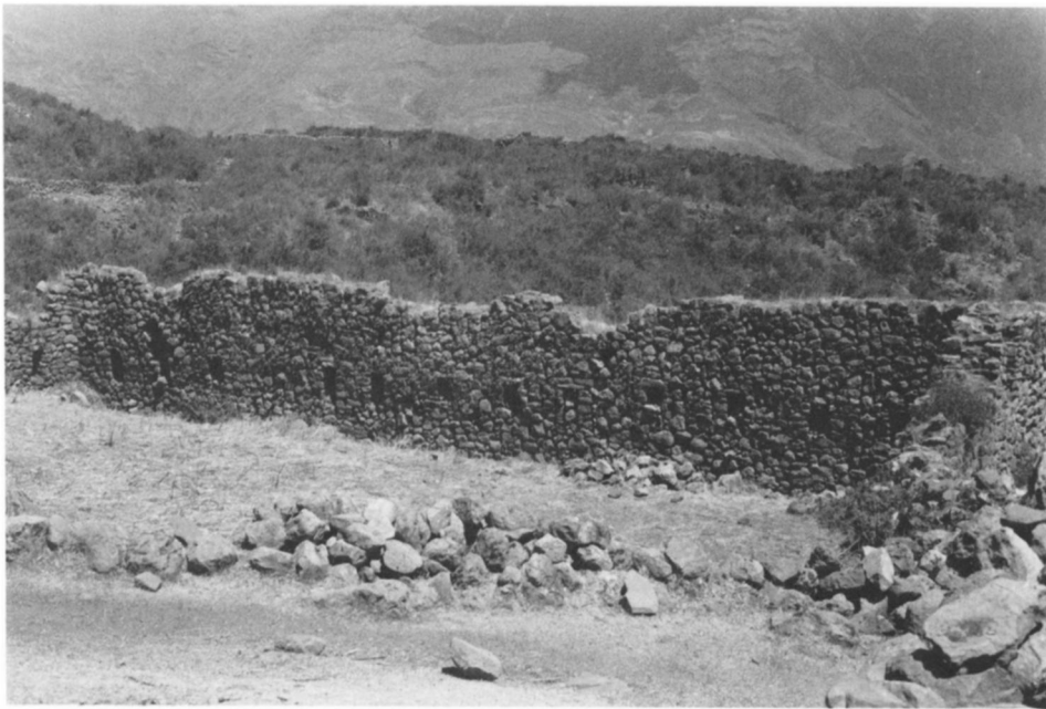
Fig. 3. Fieldstone wall of the great hall at Tipón, a royal estate near Cuzco (author).
