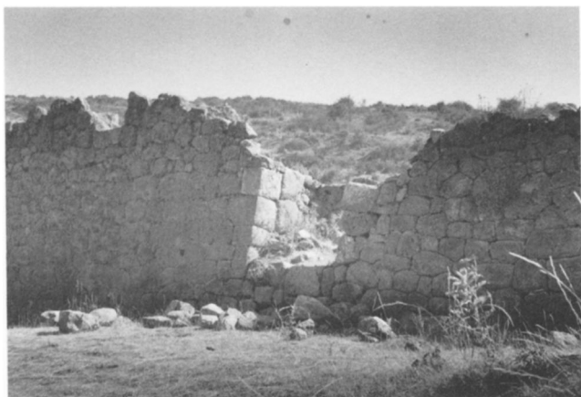
Fig. 17. Front wall, Building 1, Rumi Wasi, with coursed doorway edge (author).
